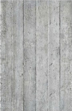
AT-GRADE EXTERIOR: VERTICAL BOARD FORMED CONCRETE
